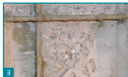
3 Renovation HB1 nechat proschnout.
